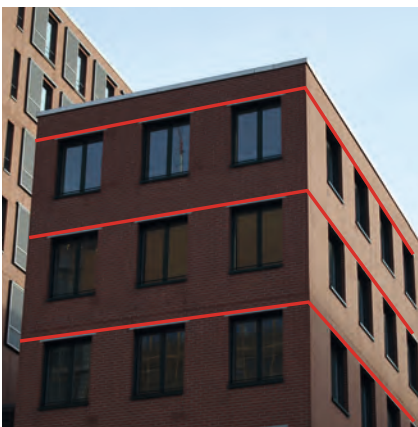
Continuous horizontal expansion joints on the same plane as the bracing, flush with the upper edge of the opening (vertical expansion joints not shown)
