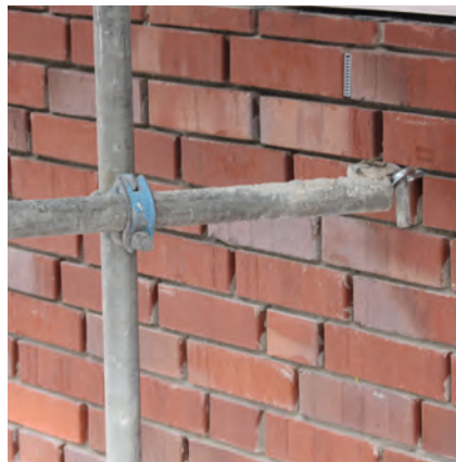
Attachment of the scaffolding to the scaffold anchor by means of a scaffolding eyelet.
