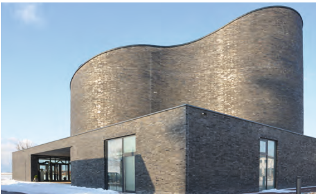
St. Marien church in Schillig: The curved shapes of the building posed a particular challenge, which was taken into account by the JORDAHL experts when planning the brackets.
