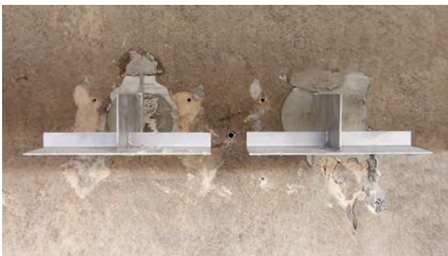
Top image: JMK+ P bracket being installed
