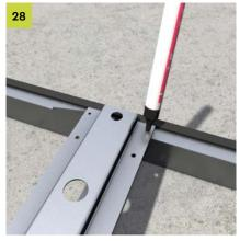
The missing fixing holes for the crossbeam must be re-drilled with a diameter of 6 mm in the cut duct section. The crossbeam can be used as a drilling template for this. A crossbeam must always be placed between two duct sections.
