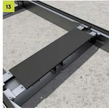
The impact sound profile is clamped centrally on the crossbeam. The drill holes for fixing the covers may not be covered.
