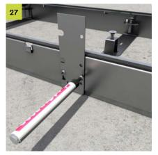
Template is required if the trunking has been shortened. Place the cut duct at the end of the uncut duct and level it to the same height. Place the template over the screws on both sides and drill holes (Ø 6 mm) opposite the screw heads. Screw the cut duct to the levelling support.
