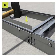
The adjusting strip can be inserted with the help of a rubber mallet.
