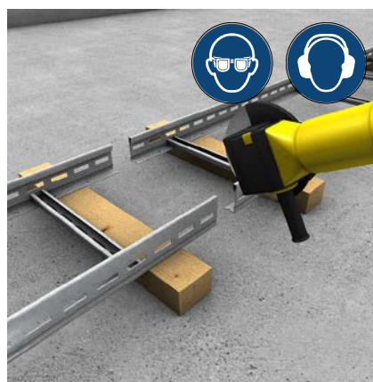
Fig. 2: Observe occupational safety measures during cutting and separating work
