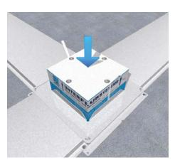
4 | Inserting the shuttering unit
