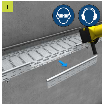
Tray extension joint (RAA) Cut out the side rail of the cable tray flush with the bottom in width B = connecting cable tray width + 120 mm, deburr and cold-galvanise.
