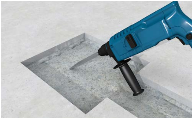
Correct any unevenness with a hand router or a caulking hammer.
