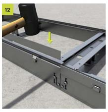
The adjusting strip can be inserted with the help of a rubber mallet.
