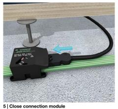
After fixing the cables close the upper case chamber and lock with a clearly audible click. If the cover does not close completely, not all screws have been tightened correctly. Attach the connecting cable with plug component to the flat cable adapter and lock it with an audible click.
