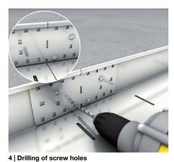
If the floor duct is shortened, drill two new screw holes in each side beam. Drill  $2 \times D = 6.5$ mm through the holes in the pre-assembled floor duct coupler, as shown.
