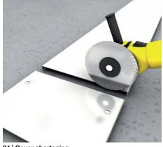
**24 | Cover shortening** If the turning bolts on the floor duct covers have been removed while shortening, fit two new turning bolts opposite to each other, if the distance between the last turning bolt and the cover end exceeds 150mm.
