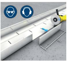
**9** | Floor duct attachment branch-piece While installing additional floor duct branch pieces produced on-site, cut out the side beam of the floor duct at a width B = width of the connecting duct + 120mm (flush to the floor), deburr and cold-galvanise.
