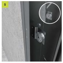
Use a 7 mm open-end spanner to attach the magnetic holder to the bolts of the base body using the nuts supplied.
