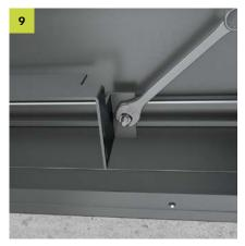
Fix the device carrier in the rail run using the nuts and hammerhead screw supplied
