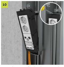
Insert the customised and connected mounting box into the device carrier. Use a slotted screwdriver to make installation easier.
