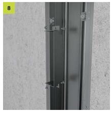
Position the device carrier according to the use and the cut-outs on the panel.
