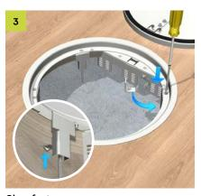
**Claw fastener**Fit the provided claw fastener with the appropriate screws in the frame and tighten them.
