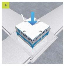
**Inserting the shuttering unit** Insert shuttering unit straight from the top into the floor box opening. Floor box and shuttering unit make one mounting unit. Mask all openings in the duct system. Apply insulation flush to duct system and to shuttering unit.
