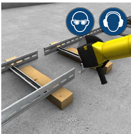
Fig. 1: Observe occupational safety measures during cutting and sectioning work.
