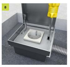
After connecting the socket, the cover plate is fixed to the frame of the floor socket again using the screws. Observe equipotential bonding.
