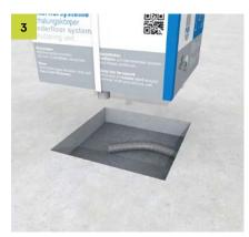
After the screed has hardened, carefully remove the formwork body using the ripcord.
