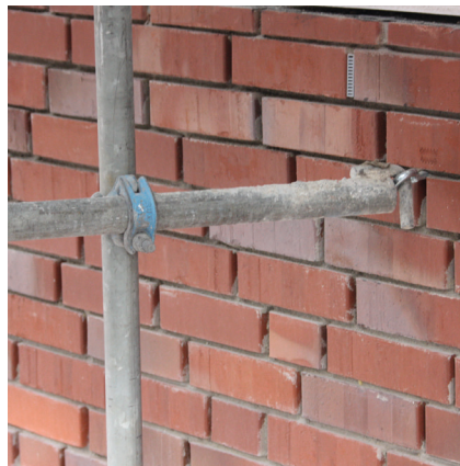
Attachment of the scaffolding to the scaffold anchor by means of a scaffolding eyelet.
