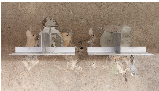
Top image: JMK+ P bracket being installed
