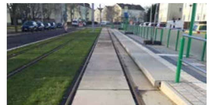
Tramway cover plates, Magdeburg, Germany
