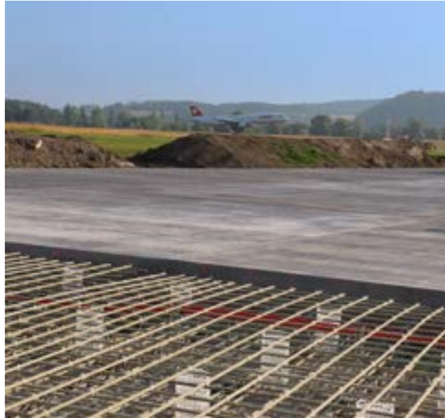
Construction of a new taxiway Zurich Airport, Switzerland
