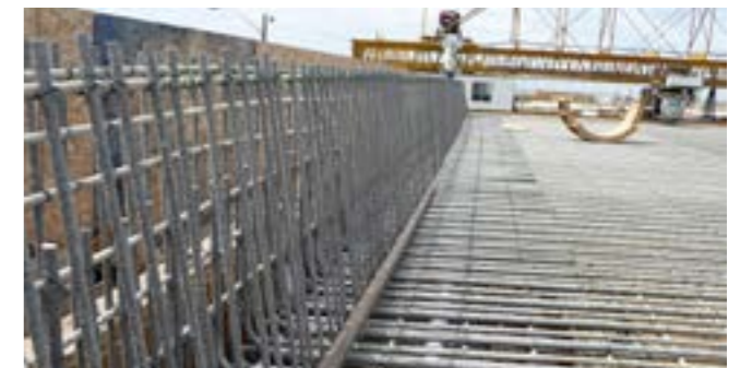
Installing FIBERNOX® V-ROD in bridge deck and concrete guard rails
