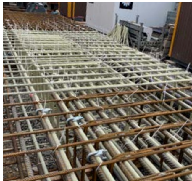
Diaphragm wall of motorway enclosure Schwamendingen, Switzerland
