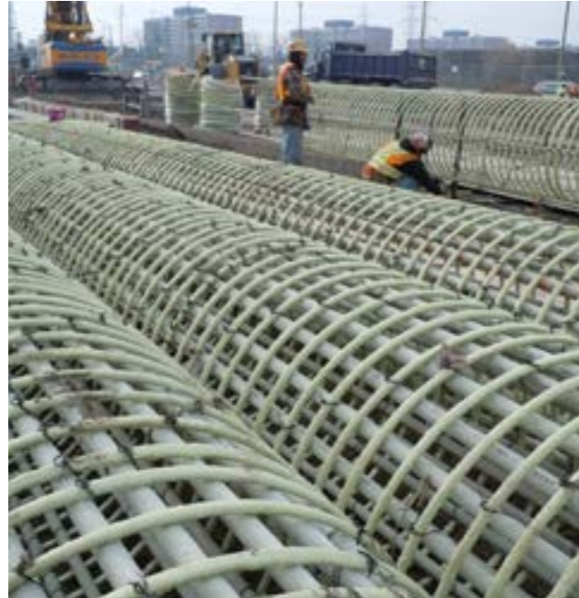
Reinforcement cages made of straight and spiral FIBERNOX® V-ROD reinforcement
