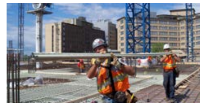
FIBERNOX® V-ROD used as a non-conductive floor slab reinforcement for new hospital construction
