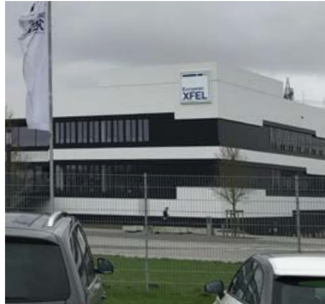
Reinforcement of the research buildings in the Undulator Hall European XFEL GmbH, Schenefeld, Germany
