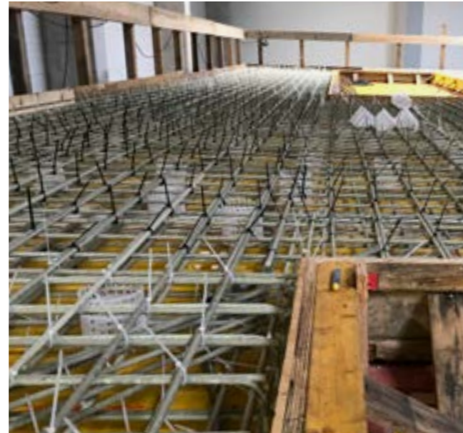
Ceiling slab reinforcement European XFEL GmbH, Schenefeld, Germany
