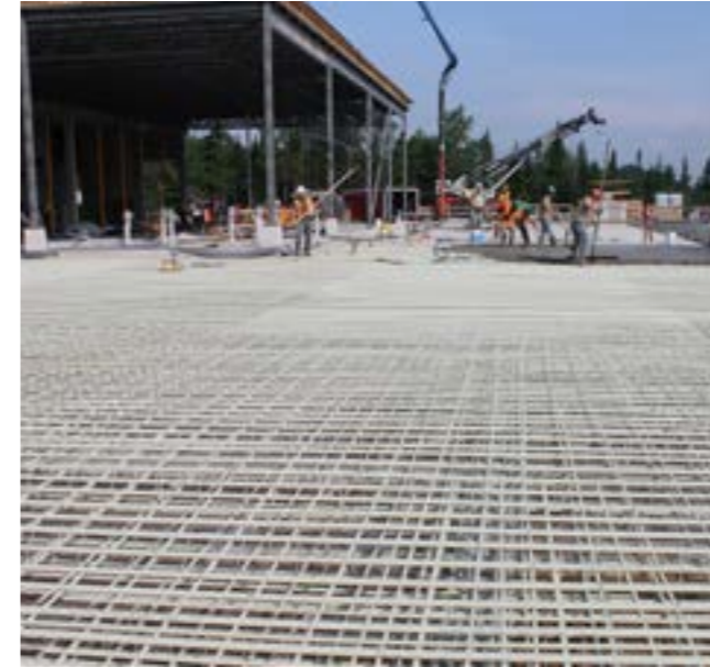
Tanks for sewage treatment plant, floor slab reinforcement Thetford Mines, Québec, Canada
