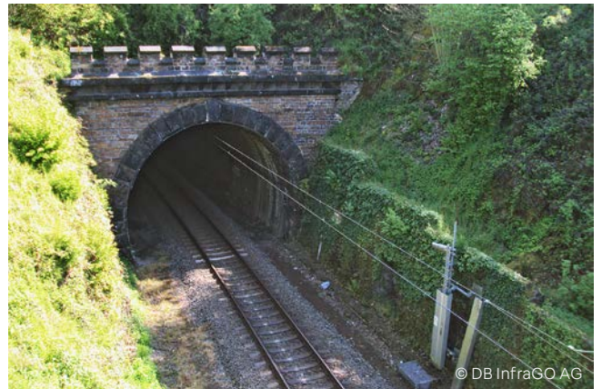
Horchheim Tunnel, refurbishment (Koblenz, Germany)
