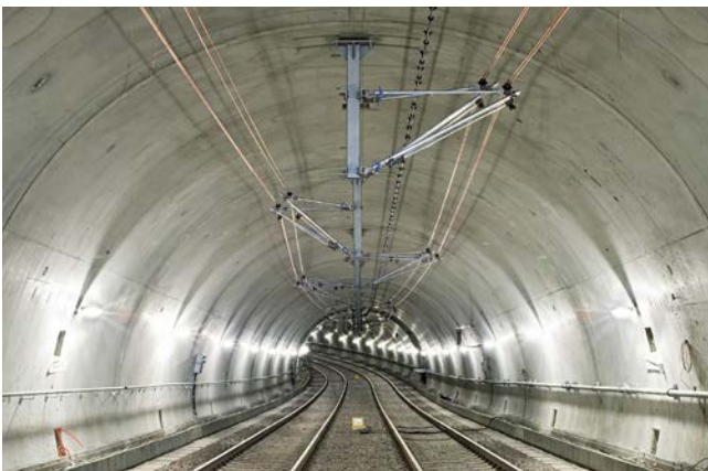
Extension of the U6 metro line (Stuttgart, Germany)
