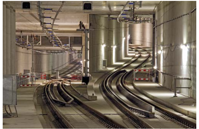
City-Tunnel (Leipzig, Germany)
