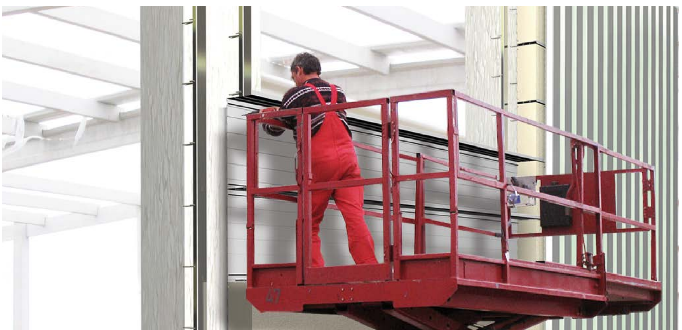
Installation of a multi-layer insulated profiled sheet metal wall.
