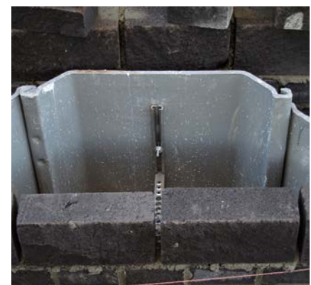
Connection of facing masonry to bulkhead wall
