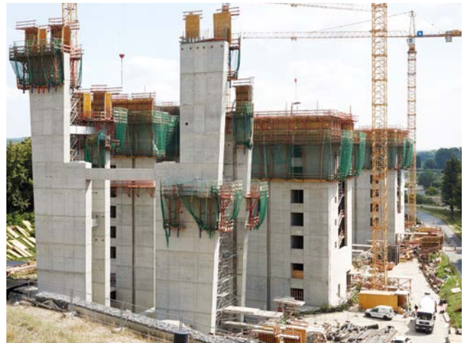
Niederfinow Boat Lift, Germany
