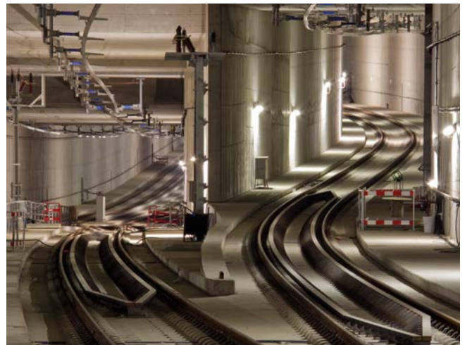
City Tunnel, Leipzig, Germany
