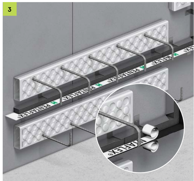
3 Next to the PENTAFLEX® Modul, nail two single-row FERBOX® rebend connectors to the formwork. Before pouring the concrete, remove the top part of the protective film from the PENTAFLEX® seam sheet.
