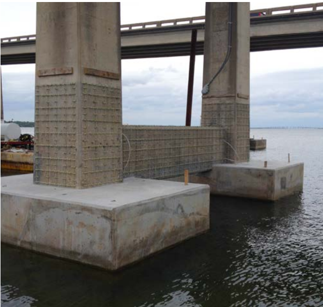
Refurbishment of bridge supports in salt water Florida, USA
