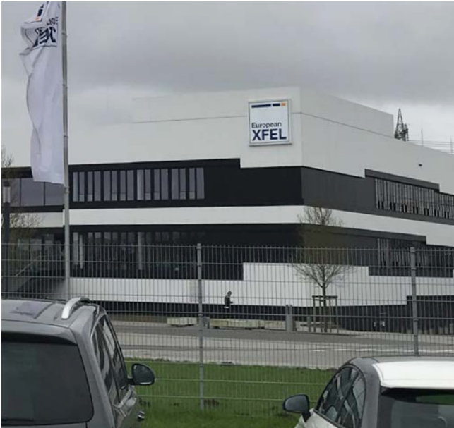
Reinforcement of the research buildings in the Undulator Hall European XFEL GmbH, Schenefeld, Germany
