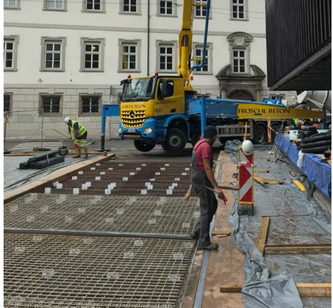
Creative concrete forecourt Haus der Musik, Innsbruck, Austria
