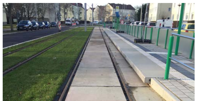
Tramway cover plates, Magdeburg, Germany
