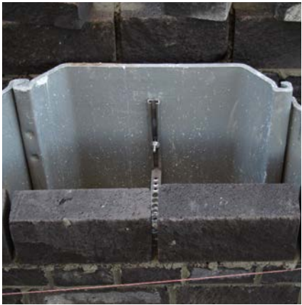
Connection of facing masonry to reinforced concrete components
