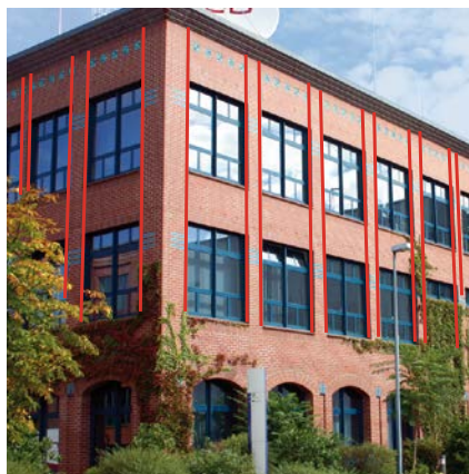
Continuous vertical expansion joints next to openings (horizontal expansion joints not shown)
