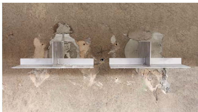
Top image: JMK+ P bracket being installed
