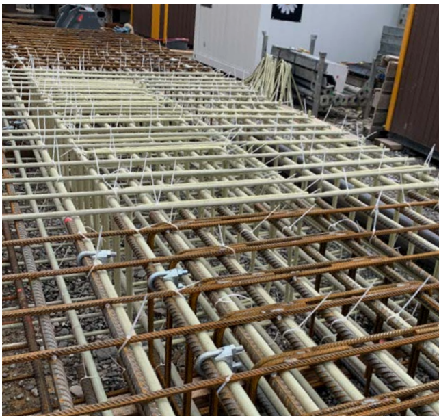
Diaphragm wall of motorway enclosure Schwamendingen, Switzerland
