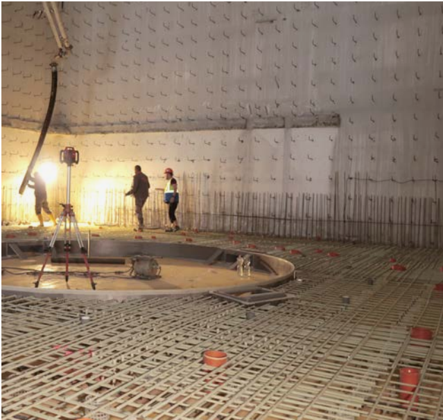
Ground slab and column reinforcement as well as punching shear reinforcement Fusion energy research project Tokamak in Prague, Czech Republic
