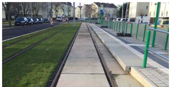
Tramway cover plates, Magdeburg, Germany
