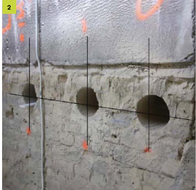
Kernbohrungen setzen – wahlweise Loch stemmen. Perform core drilling – optionally chise out the hole.
