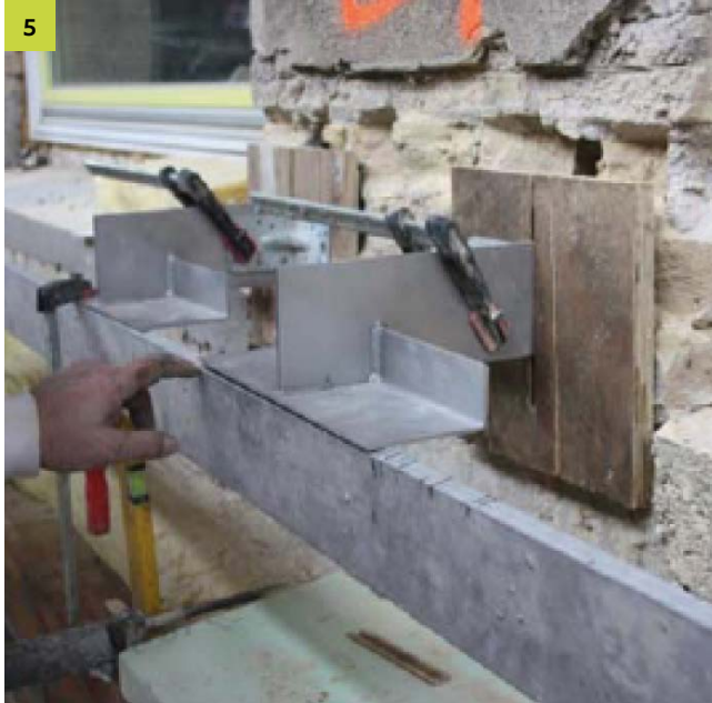
Konsole fein ausrichten (horizontal) – Schalenabstand prüfen (Tiefe). Align console precisely (horizontally) and check the shell spacing (installation depth).
