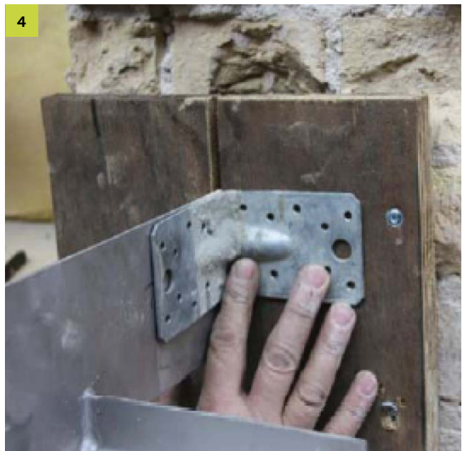
Winkelverbinder (A4) als Justierhilfe am Schalbrett befestigen. Attach angle joint (stainless steel) to the formwork board as an adjustment aid.
